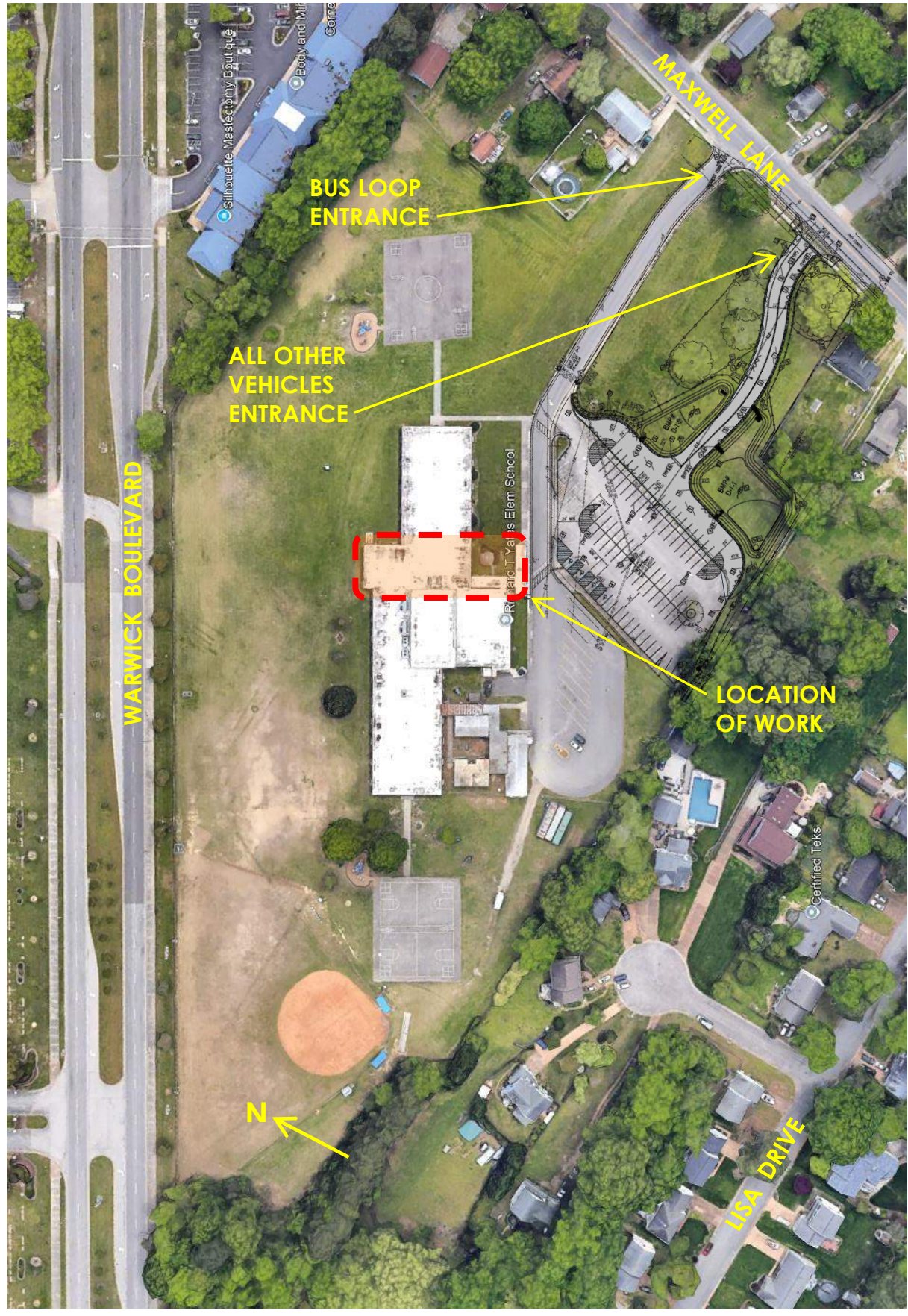
AERIAL VIEW: YATES ELEMENTARY SCHOOL (Not to Scale)
