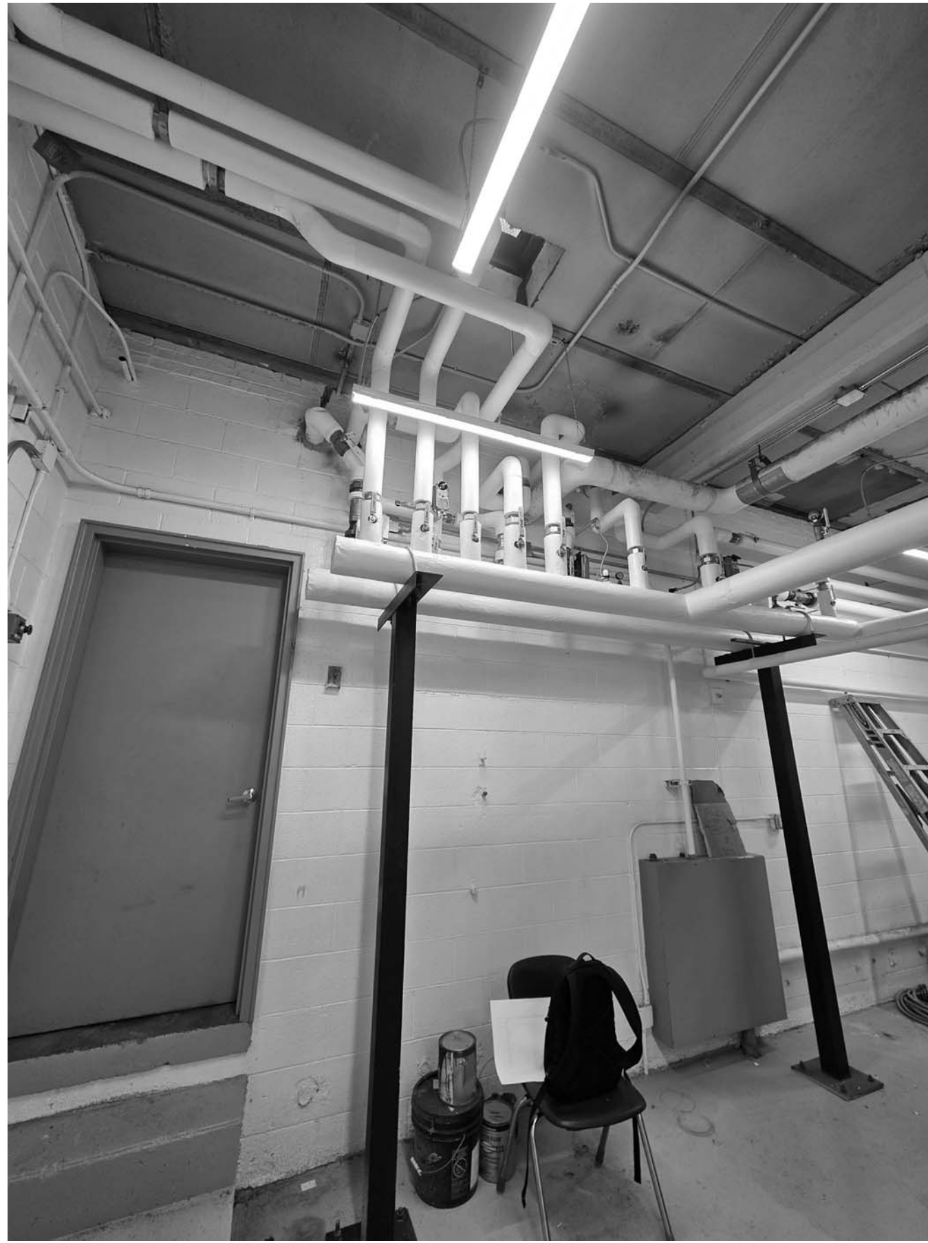
P5 PIPING AND MECHANICAL EQUIPMENT REMOVAL PHOTO MD102 NOT TO SCALE
