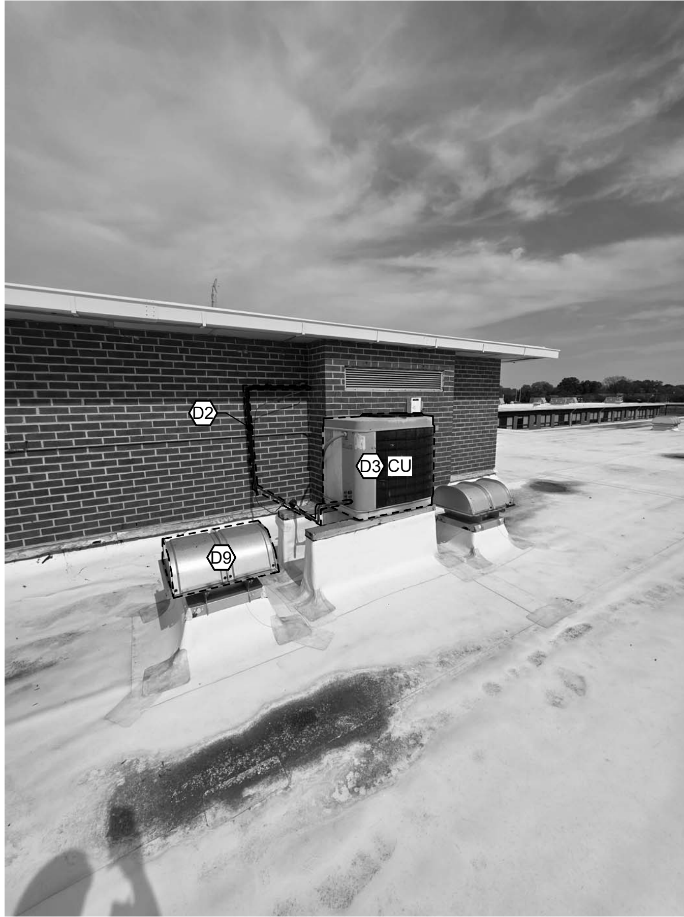
P4 CONDENSING UNIT REMOVAL PHOTO MD102 NOT TO SCALE
