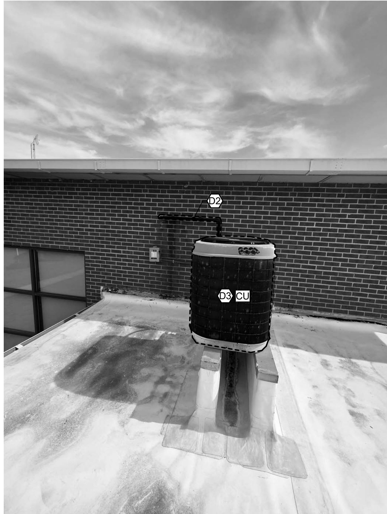
P2 CONDENSING UNIT REMOVAL PHOTO MD102 NOT TO SCALE
