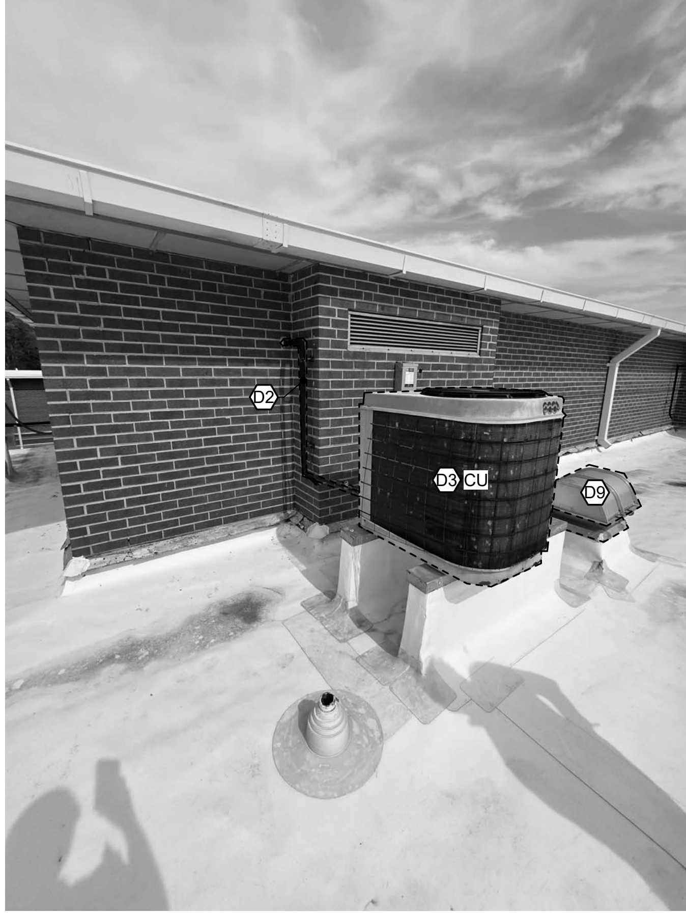
P3 CONDENSING UNIT REMOVAL PHOTO MD102 NOT TO SCALE
